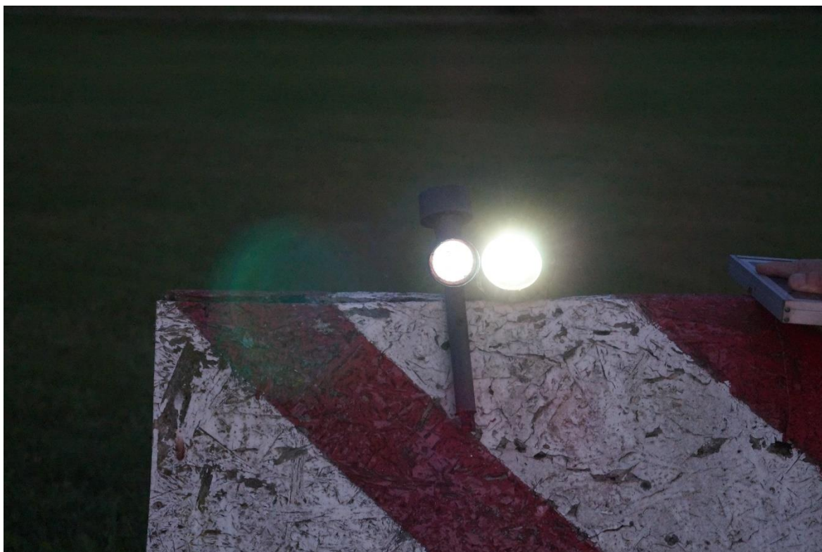
Fig. 7 Solar lamps at the end of runway
